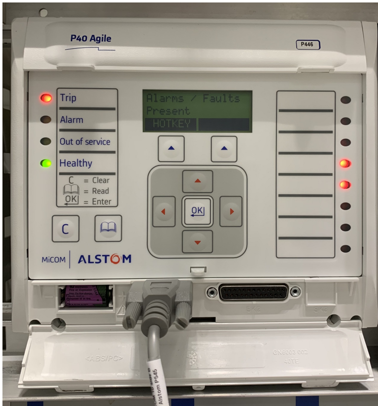
Figure 4.1: MiCOM Alstom Distance Relay P446
