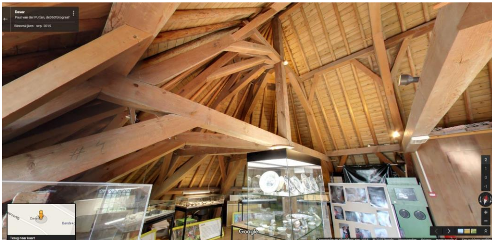
Figure 3.30 Restored roof structure of 't Huys Dever. Source: https://goo.gl/maps/SohZsBspQwM2
