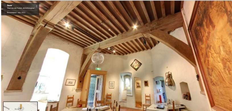
Figure 3.32 The restored floor structure of 't Huys Dever. Source: https://goo.gl/maps/SohZsBspQwM2
