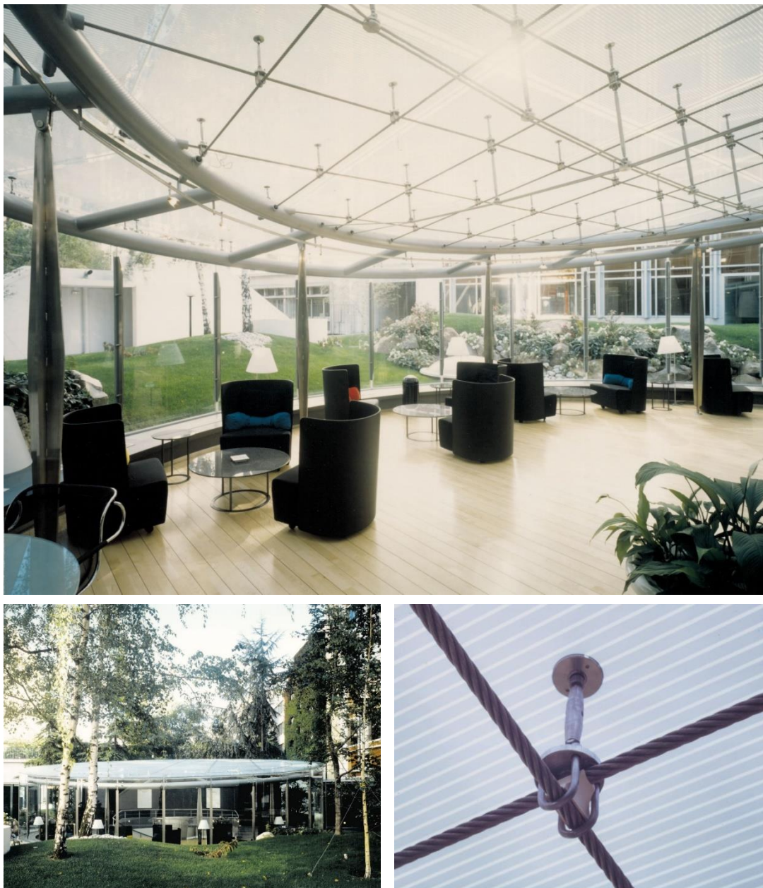
Figure 5.15 The cable/truss roof structure of Rotunda reception building. Source:(Schittich et al., 2007)
