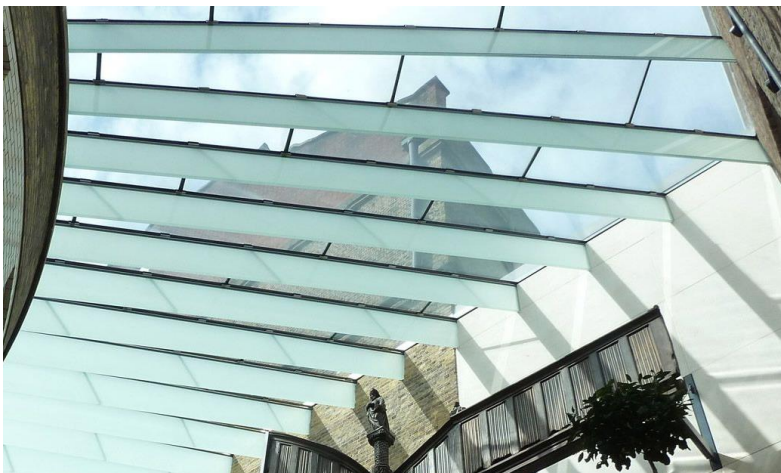
Figure 5.9. The structural glass roof structure of the Victoria & Albert Museum. Source: http://www.octatube.nl/projecten/4/victoria-albert-museum-daylit-gallery/
