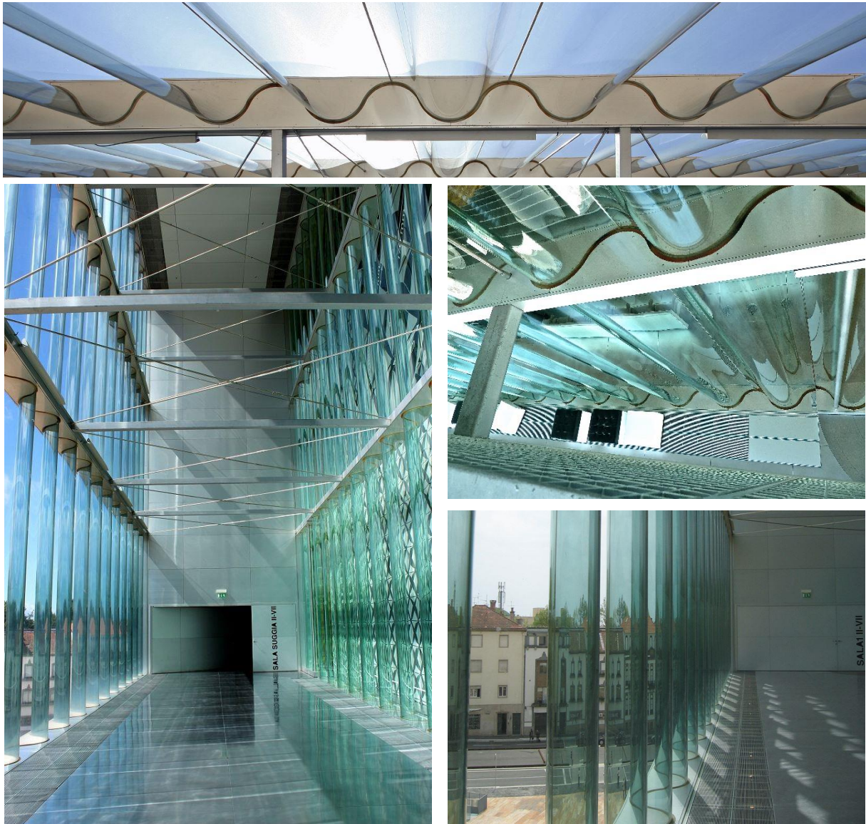
Figure 5.19. An overview and close-up of the corrugated glass façade in Casa da Musica.
