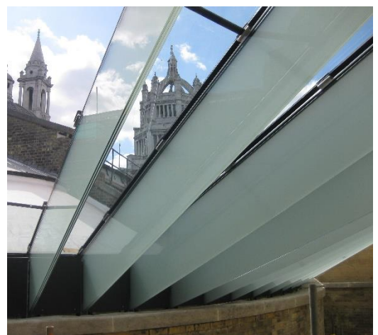
Figure 5.9. The structural glass roof structure of the Victoria & Albert Museum. Source: http://www.octatube.nl/projecten/4/victoria-albert-museum-daylit-gallery/
