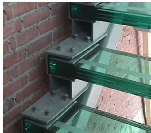
Figure 4.22 A clamped glass stair tread. Source: (Nijse, 2013)
