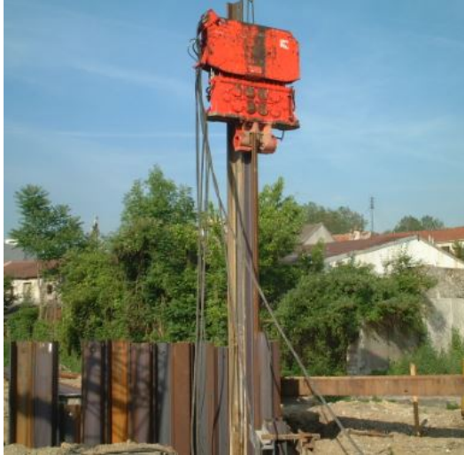
Figure 1.2: Pile driving system
