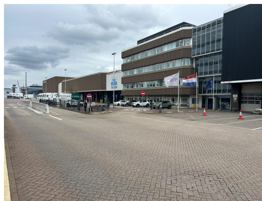
Figure 1.5: Corridor from FB2 to FB3
