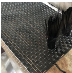
(a) Carbon fiber anchors inserted into concrete
