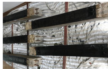
(c) Finished RC beams reinforcement.
