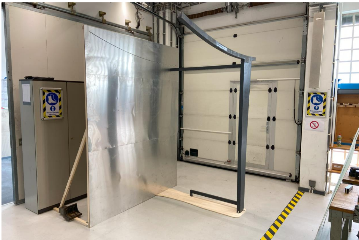
Fig. 8.1: Construction of wooden framework for demonstrator
