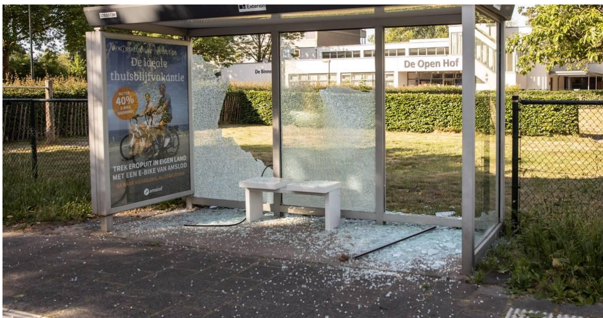
Fig. 7.1: Example of vandalism at bus shelters (Huurdeman, 2020)
