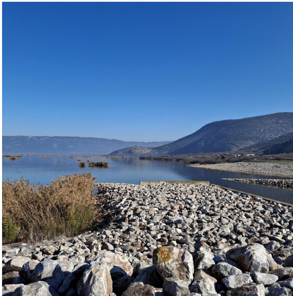
at the floodgate Lake Karla, December 2024
