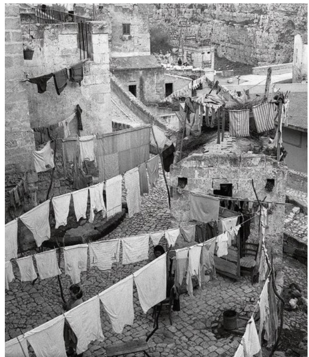
Figure 1. Photograph of hanging laundry in the Sassi, unknown. Reproduced from www.wikimatera.it
