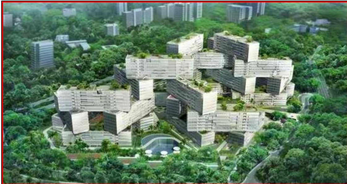
Figure 6. Complex and innovative development design (Source: The Interlace)
