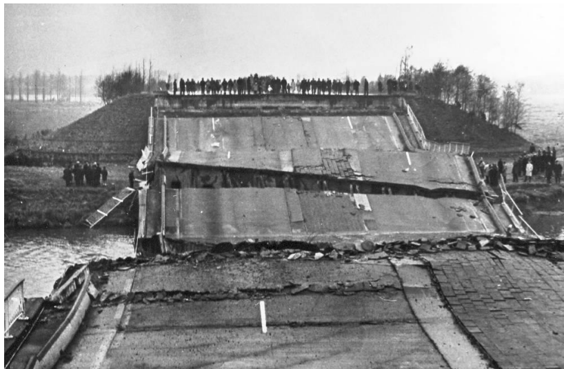
Figure 10.6 This bridge over the highway 'Boudewijn' in Pulle collapsed (1966) due to erosion of the east bank in the vicinity of the pile foundation at the side of the canal Nete
