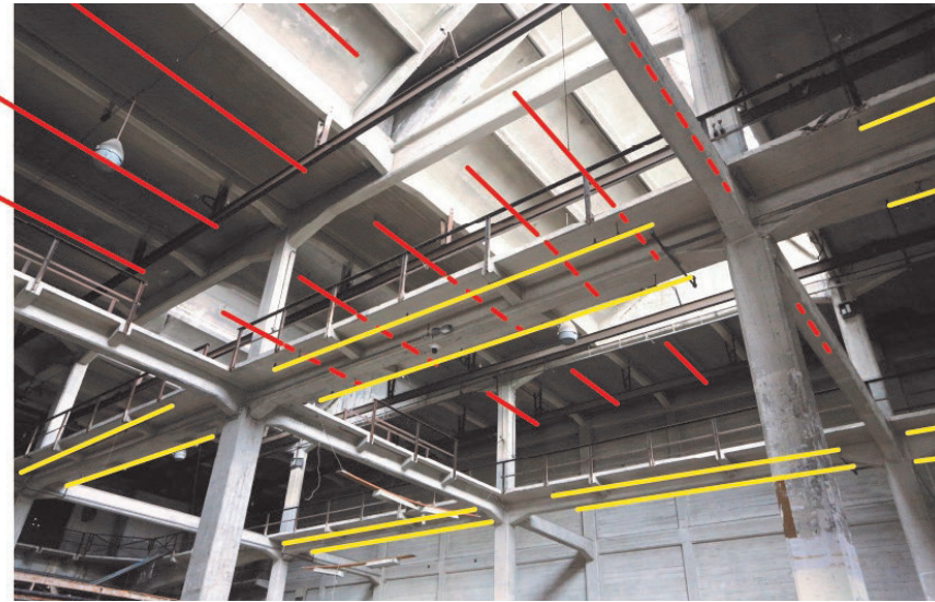
fig1. Sprinkler rails are placed on 2 different heights in the building.
