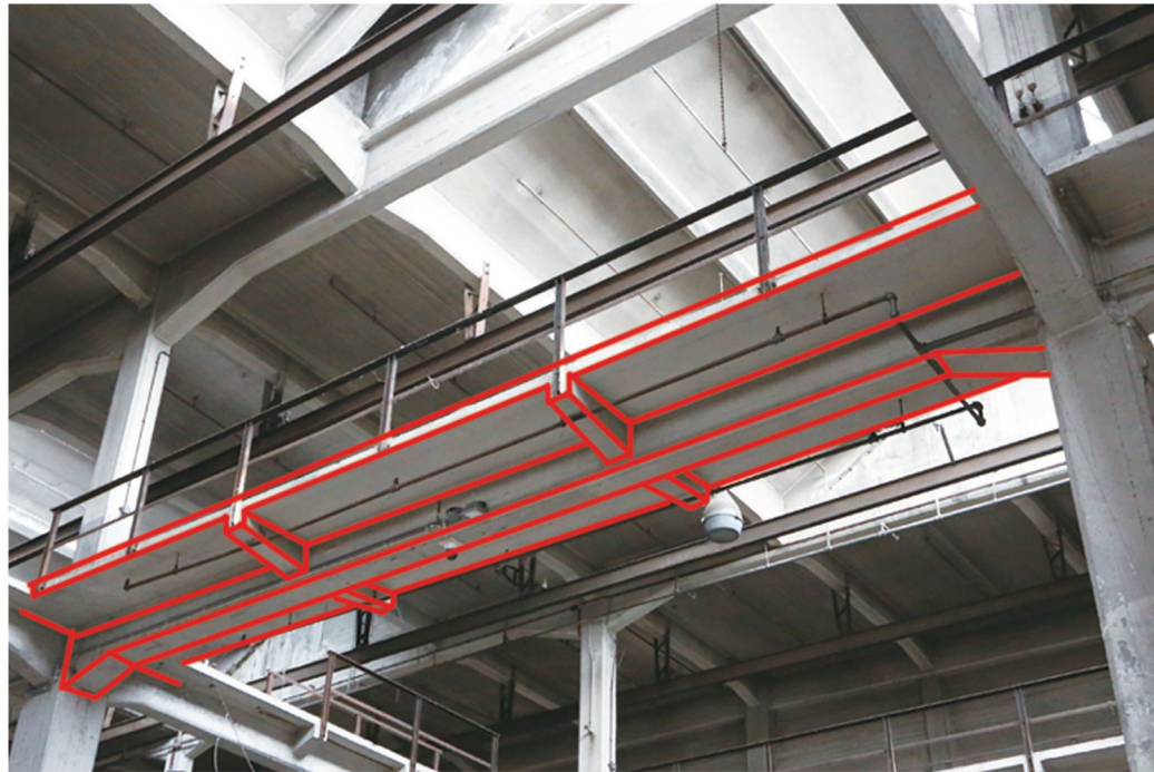
fig1. The walkway with secondary beams and steel hand rails.(marked in yellow)
