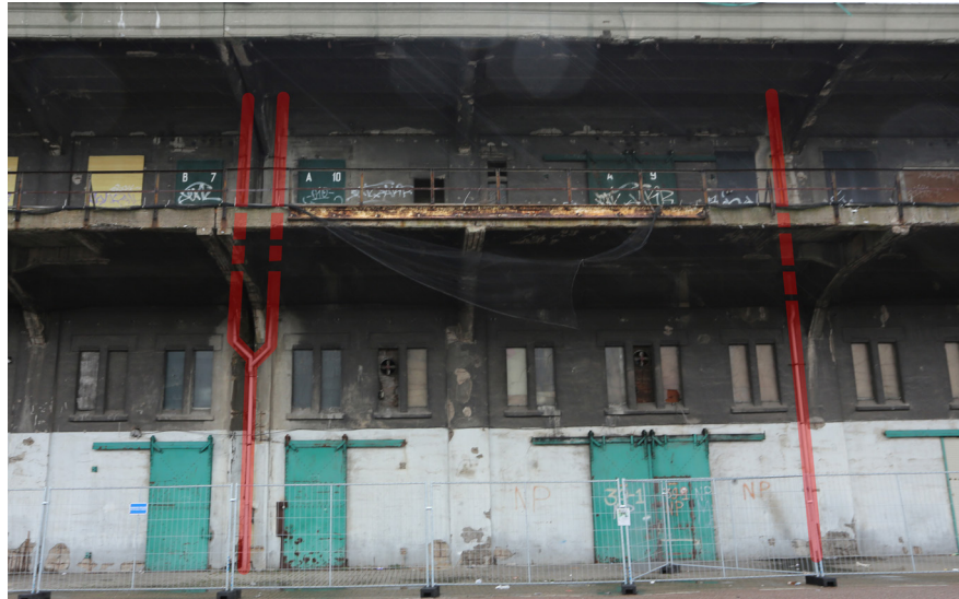
Drainage pipes shown on the facade.
