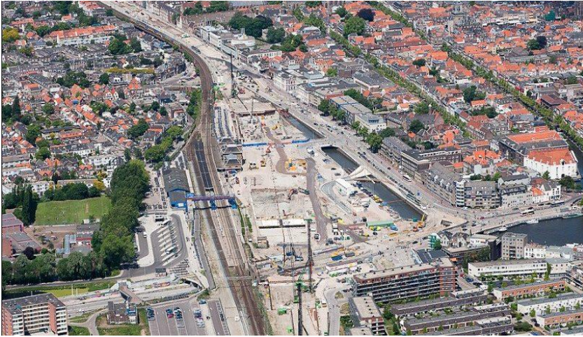
Figure 9. Construction area – Spoorzone Delft
