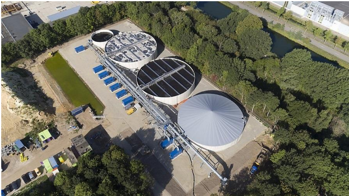
Figure 8. Water treatment plant in Weert
