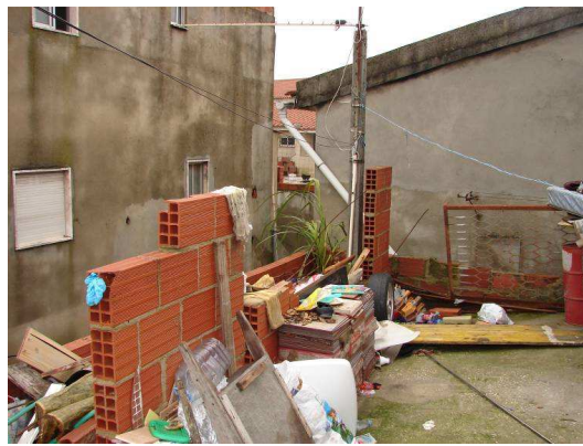
Figure 5. General appearance of a flat roof, without thermal insulation, waterproofing or any coating.
