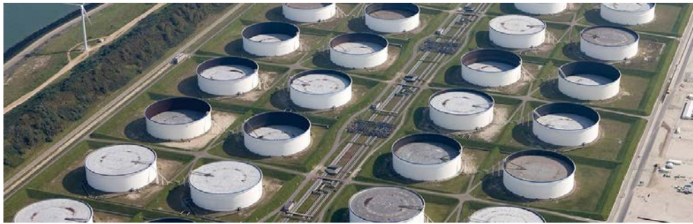
Figure 5.6: Containment bunds around oil storage tanks at the Maasvlakte Oil Terminal in the Port of Rotterdam (from www.vopak.com , Maasvlakte Olie Terminal (Rotterdam) by Vopak. Copyrights 2021 Royal Vopak.).
