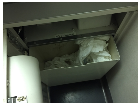
Fig.5.15 Bin full of waste paper
