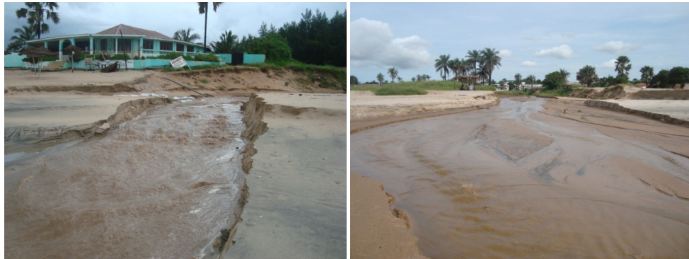
Figure 3-19: Gaps in the beach due to drainage problems
