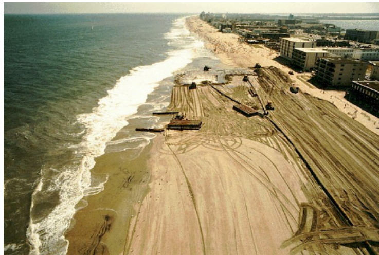
Figure 7-6: Beach nourishment in progress
