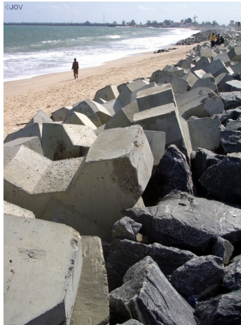
Figure 7-5: Revetment along a coast
