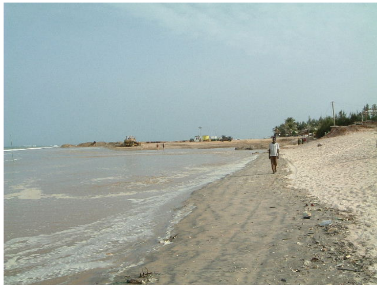
Figure 2-9: Construction of Kololi Beach
