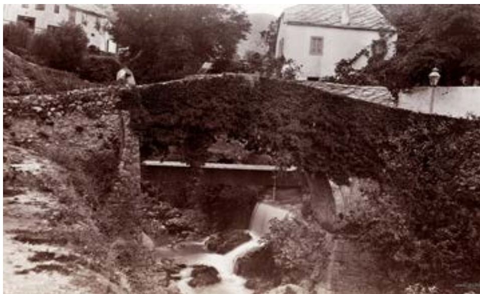
Picture 21: The bridge over the Radobolja
