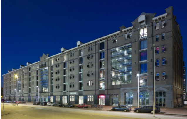
Figure 11: The Sint Jobsveem in Rotterdam (Mei architects, n.d.).
