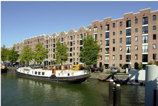
Figure 12: The Entrepotdok in Amsterdam (Architectuurgids.nl, n.d.).
