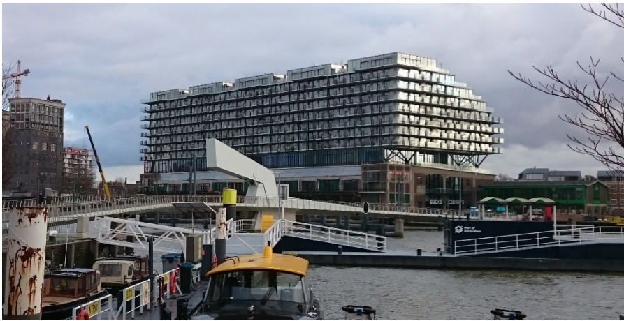
Figure 2: Fenix 1 warehouse after transformation (own photo, taken during CSI course).
