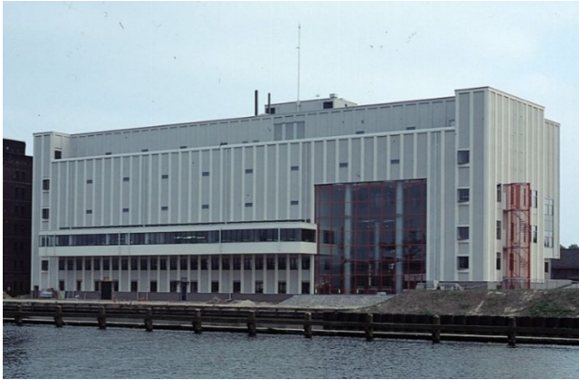
Figure 14: The Former Koning Willem I warehouse in Amsterdam (Atelier Pro, n.d.).
