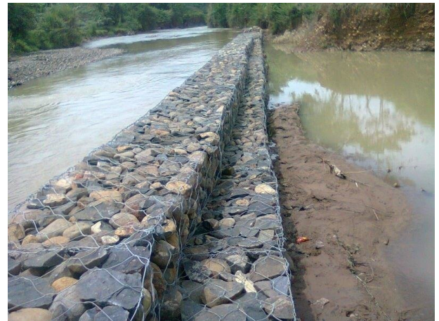
Figure 5.8: A gabion wall placed parallel to the stream channel, preventing bank erosion (Apriyono et al., 2019).
