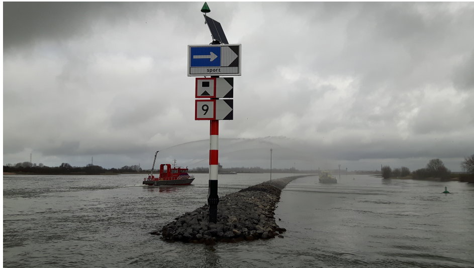
Figure 1.1: Longitudinal training wall in the Waal river (HF Midden Nederland, 2016)
