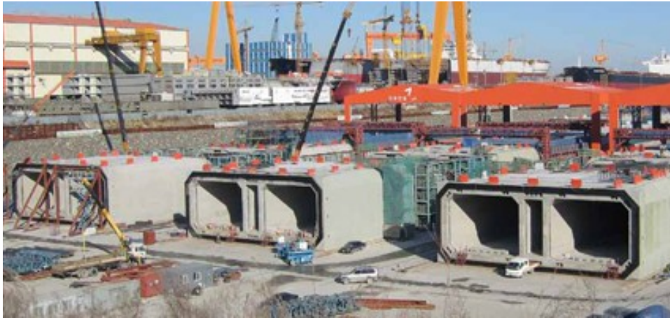
Figure 1.2 - Elements of an immersed tunnel [Ref Image 2]
