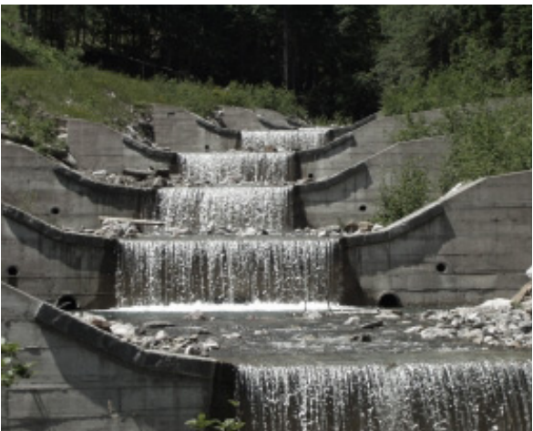
Figure 132: Drop structure in torrent Source: www.biberberti.at
