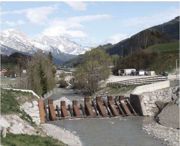
Figure 131: Barrier structure in the torrent 'Leoganger Ache' Source: Author
