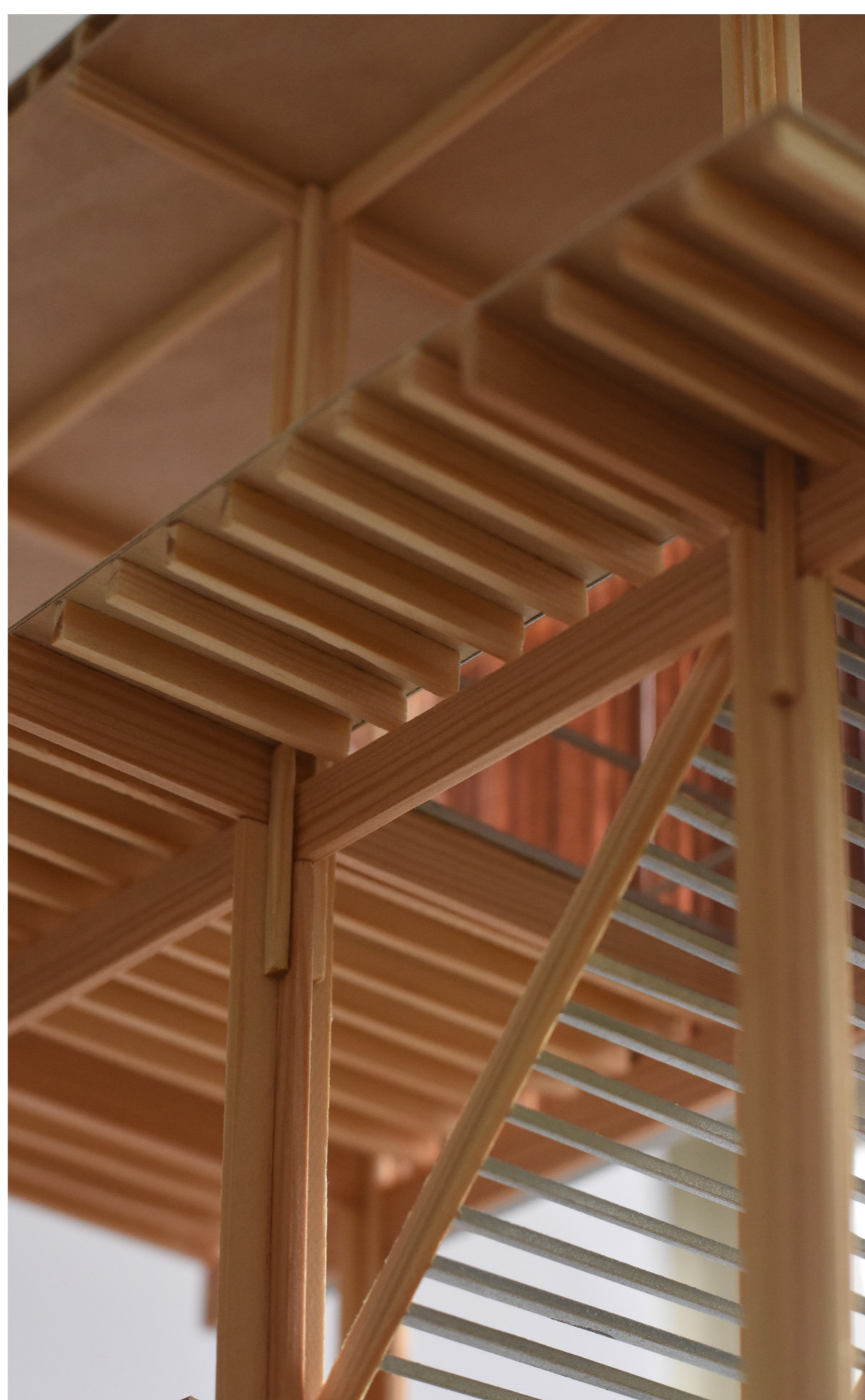
Galvanized steel baluster (10 mm steel rod, 80x30 UNP) Squared columns 4 pieces (60x60) Cross columns (400x400, flange widthness 80mm) Primary beams (80x400) secondary beams (80x200)
