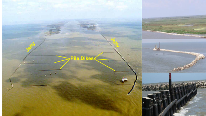
Figure A.5: Southwest Pass Infrastructure Left: Southwest Pass Jetty Structure. Top right: Foreshore Rocks. Middle right: Jetty Structure, Down right: Pile Dikes. Source: [66]
