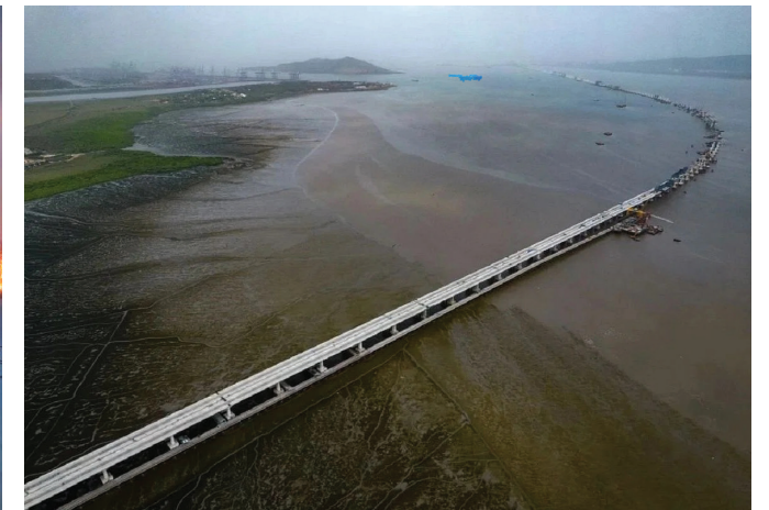
Figure 87. An actual visual of the bridge under construction captured in September, 2022. Showing its material impact on the landscape. Bridge due for completion in November 2023. Image Source : @cbdbhage/ Twitter
