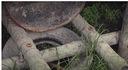
Fig. 118: Used tyres as sub-structure
