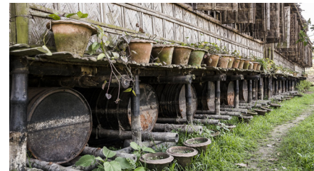
Fig. 120: Used steel drums as floating system
