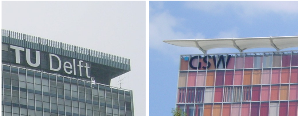
Figure 30 Influencing of the drag of a building by changing the separation velocity. Left: building of Delft University of Technology, The Netherlands. Right: building of GSW, Berlin, Germany.
