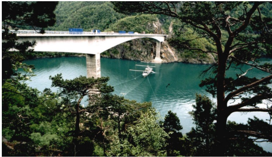
Figure 1.2: A bounded wave simulator suspended under a bridge [7]
