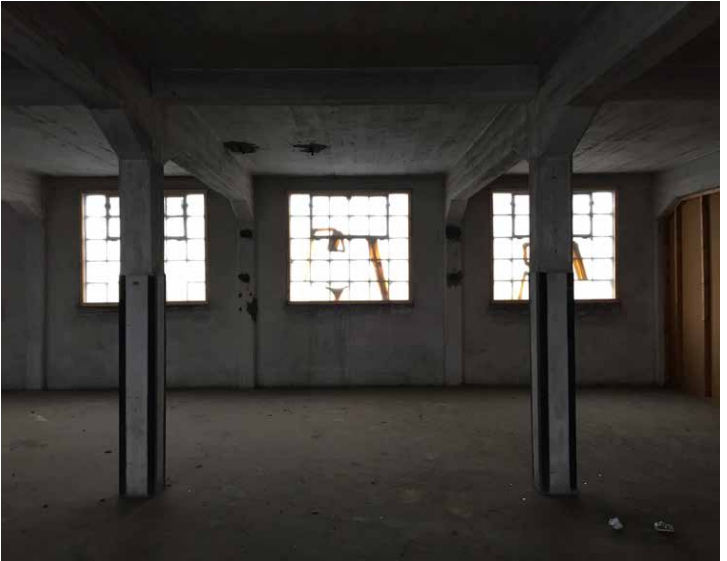
Rational structure from the second phase in concrete skeleton and masonry infill, there is stucco applied in the inside of the masonry infills from the third floor to the fifth floor.
