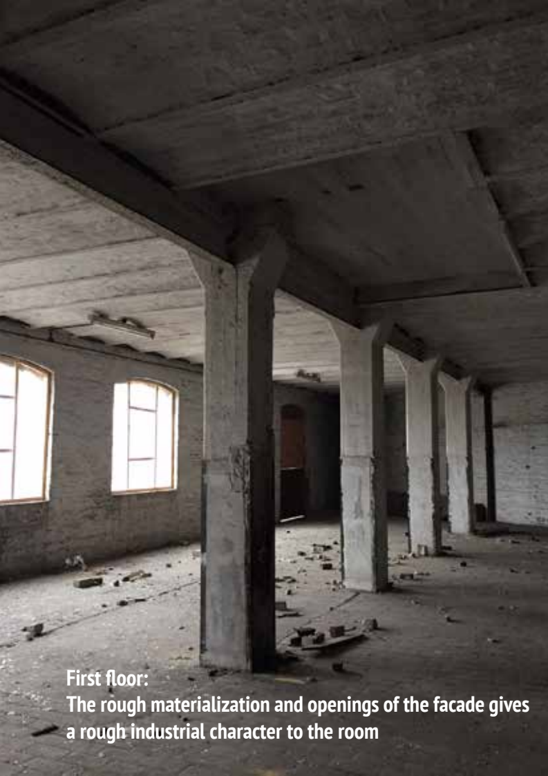
The structurally smelted room: Two different structures, Masonry walls and concrete skeleton is most visible in the second floor
