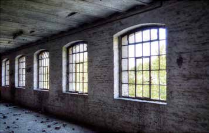
Cast-iron rectangular windows with a rounded top and have a windowsill of Namur stone from the first phase
