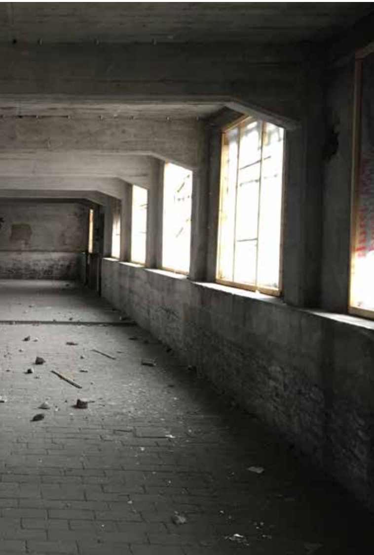
Third floor: Reinforced concrete structure with openings in the west and east facade which gives a rational character to the room
