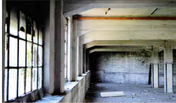
Interior space of the second floor of the Brikkengebouw showing the increased facade above the floor from the first phase where might have been a wall plate
