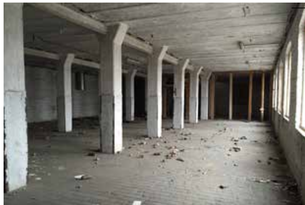
Inner-space brick hall: concrete columns and steel beam structure
