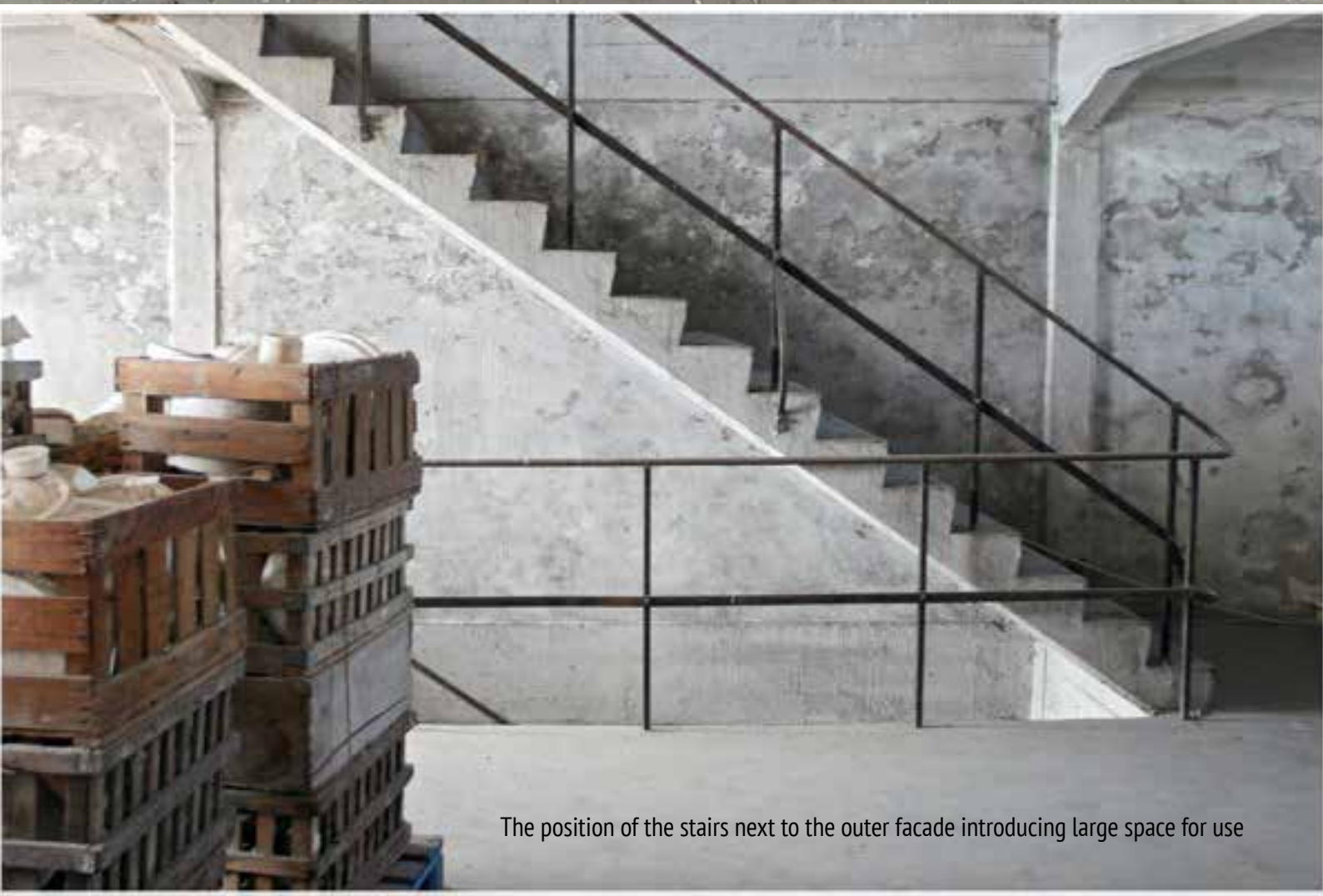
Interior photo of the building showing the stairs from the first phase void which are filled with concrete
