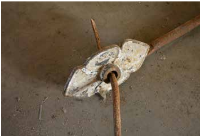
Leaf wall anchors from 1875 as an structural ornamented decor
