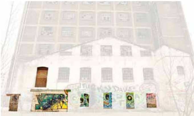
Rough crafted appearance: The windows of the ground floor are bricked completely and some big openings due functional reasoning is made
