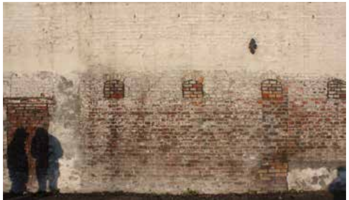
Masonry wall of the first phase with cross-bond brick construction and some small openings for ventilation
