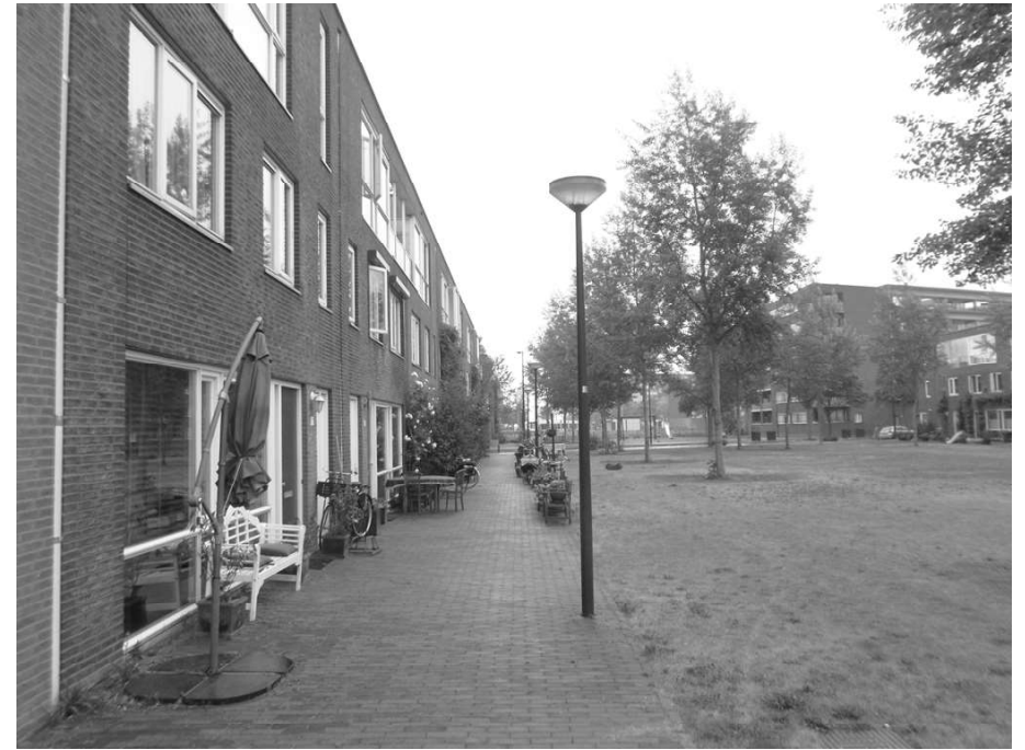
Figure 23: Streetvista of IJburg block 44a's South-East side.
