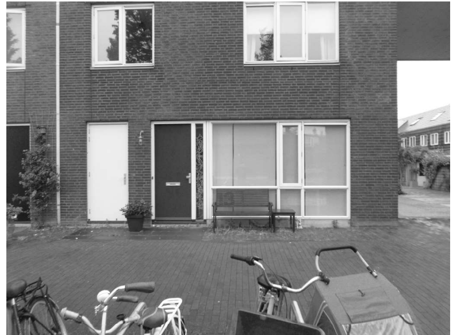
Figure 47: House facade on the North-West side of Block 44a, current situation.
