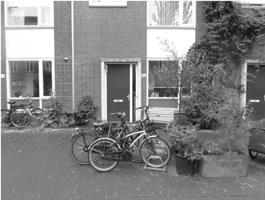
Figure 46: House facade on the North-East side of Block 44a, current situation.
