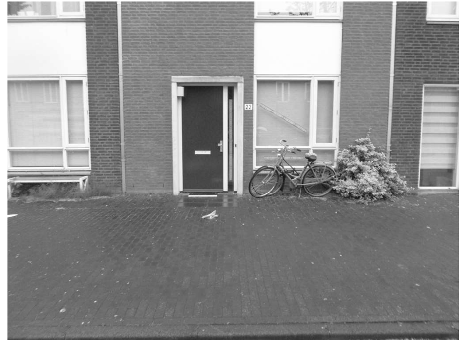
Figure 45: House facade on the North-East side of Block 44a, current situation.
