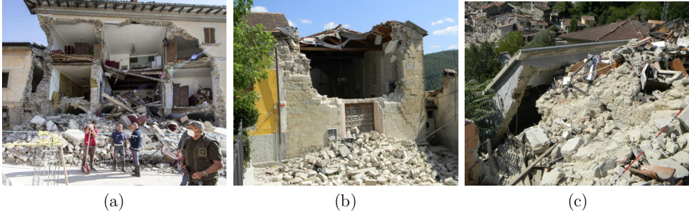
Figure 1.1: (a) Total out-of-plane wall collapse of a building after the Emilia earthquake (2012); (b) local out-of-plane collapse of a gable after Central Italy earthquake (2016); (c) total collapse of a house in which timber diaphragms were substituted with concrete slabs after L'Aquila earthquake (2009).
