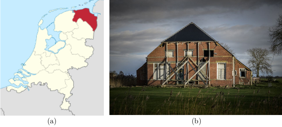
Figure 1.2: (a) The region of Groningen in the Netherlands; (b) building with structural damage after the numerous induced earthquakes taking place in the region.
