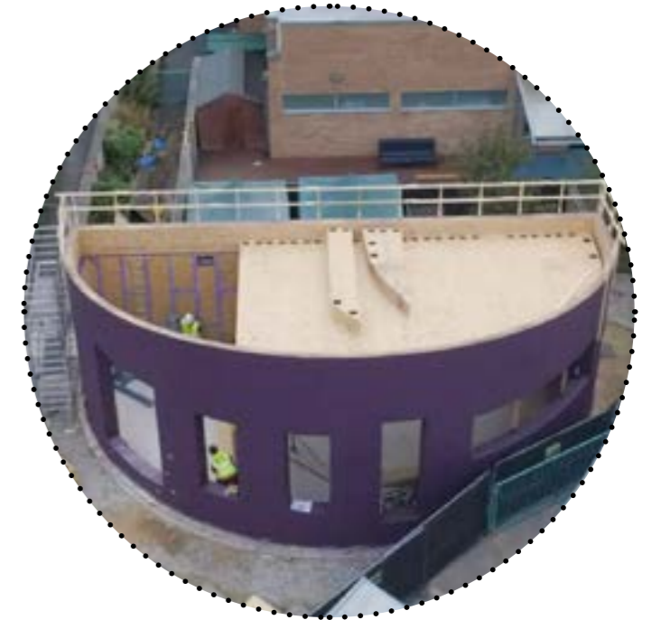
04.SPRAY AIR TIGHT LAYER / ADDITIONAL STRUCTURE FIRE PROOFING
