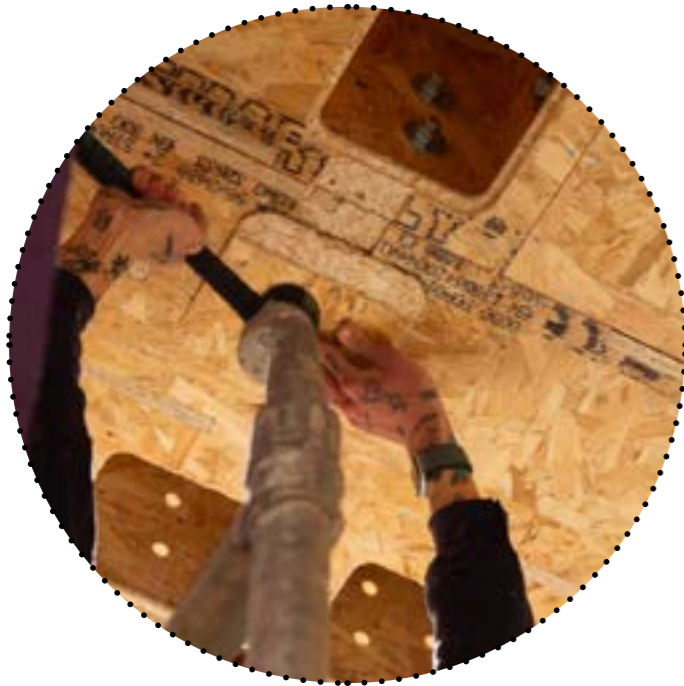
01.JUNCTION DETAILING STEEL ROD JOINTS
