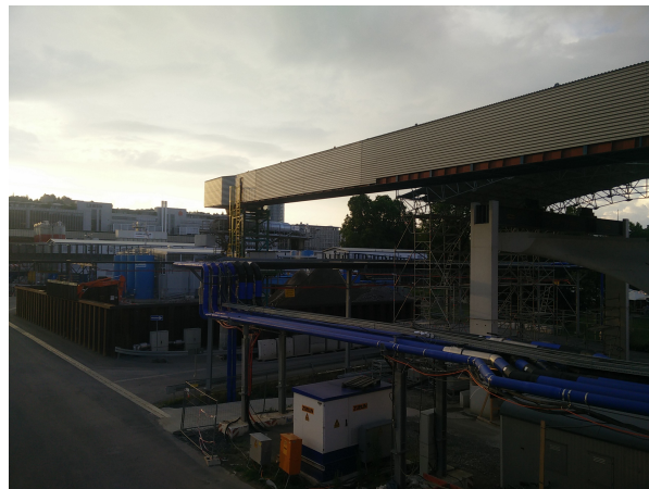
Figure 6.2: Fully enclosed conveyor in urban area. [54]
