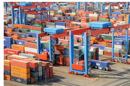
Figure 2-4: RMG cranes serve the AGVs in the yard.
