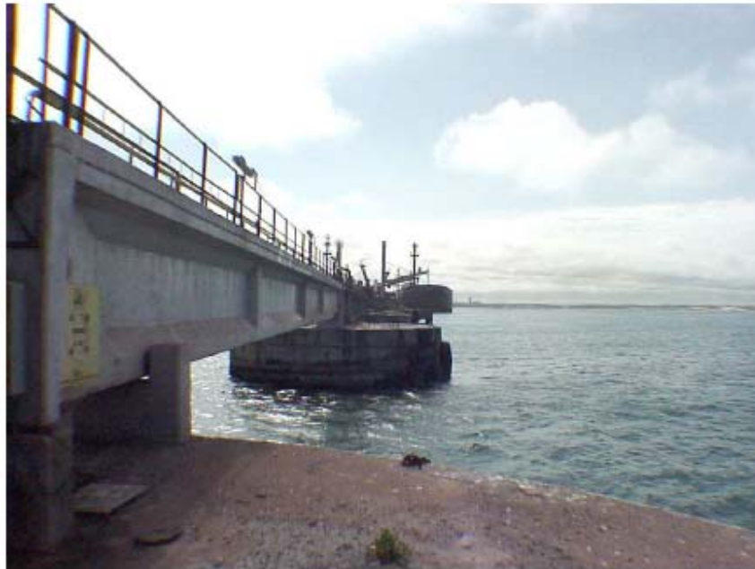
Figure A.1 Photograph showing the jetty construction
