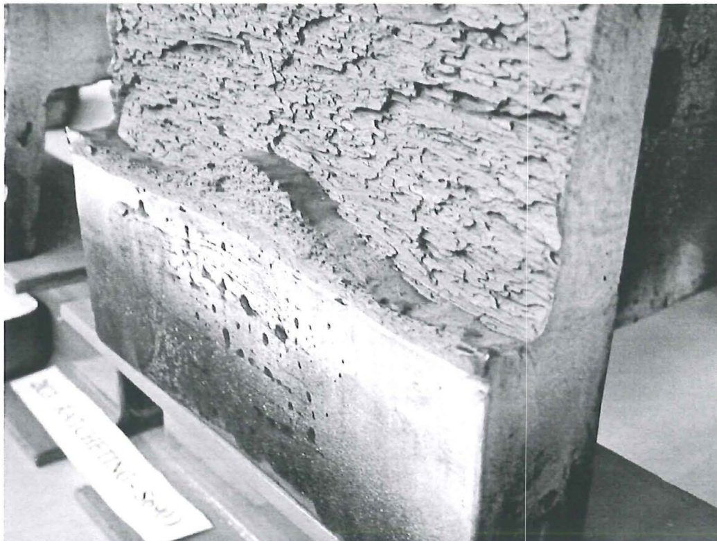
Figure 2C3-10 a/b: Observed failure
