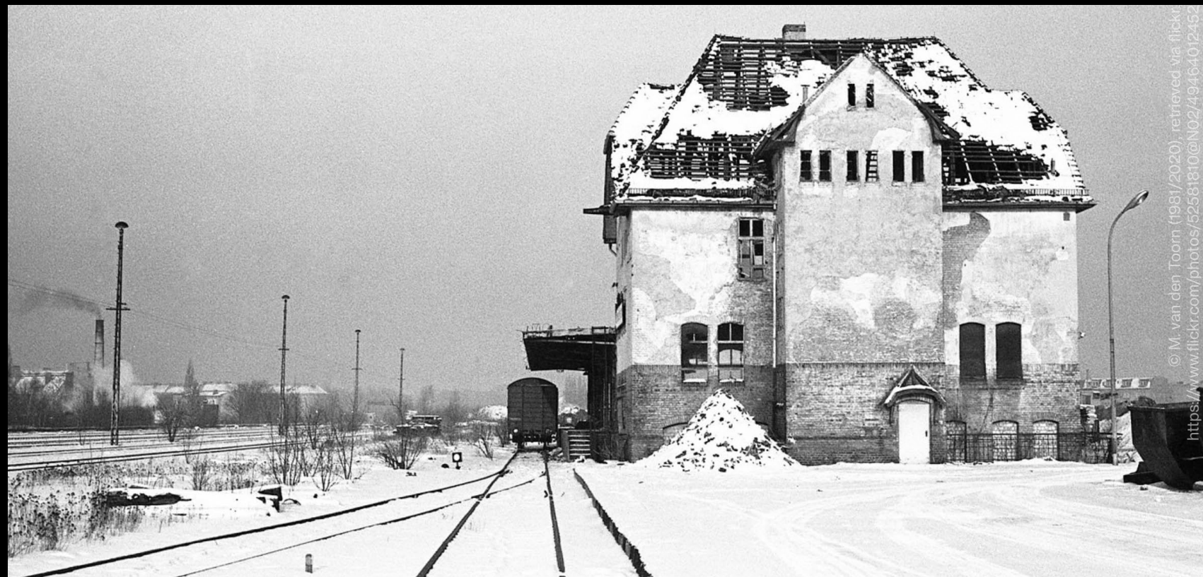
Winter 1981 Due to the proximity of the border wall, the station in West Berlin was almost unused during the separation of Berlin. It experienced a revival in the 1990s before being demolished to make space for the sand deposit.
