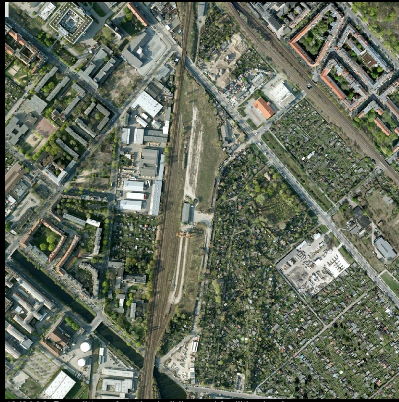
10/2009 Demolition of station building and facilities begins.
