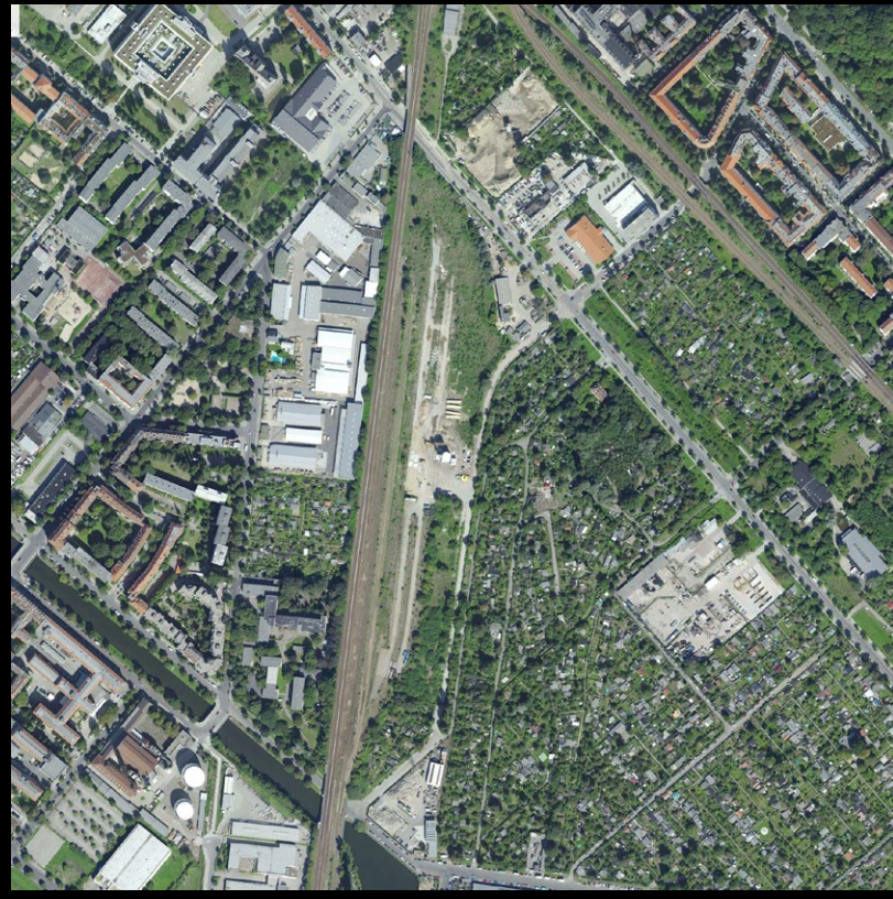
09/2010 Demolition is finished, HeidelbergCement sets up a cement plant on the plinth of the former freight station building.
