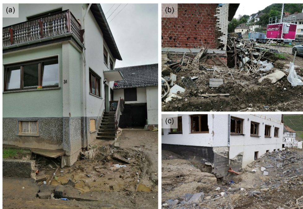
FIGURE 4 Scour at various buildings corners in: (a) Schuld; (b) Altenahr; (c) Marienthal.
