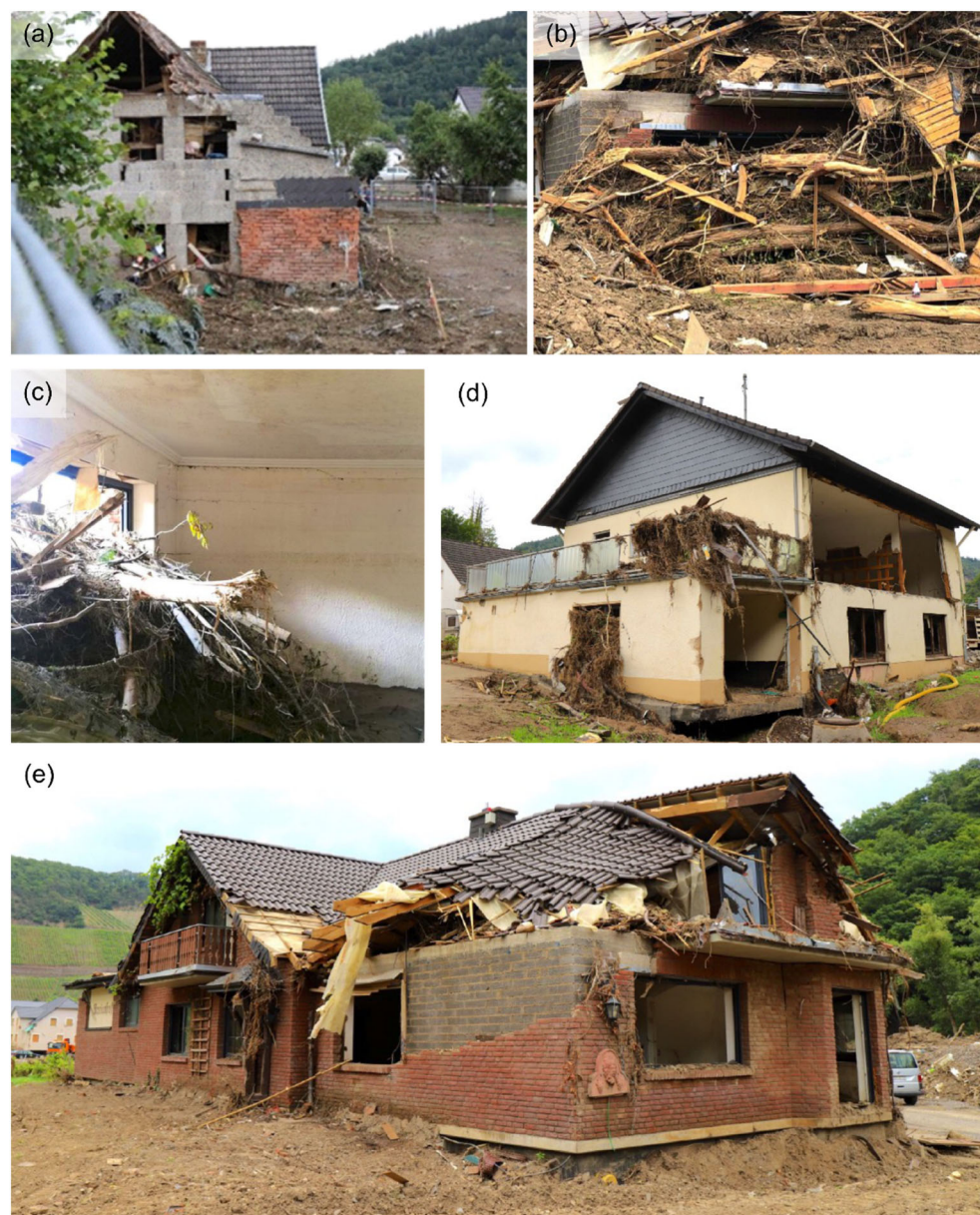
FIGURE 15 Photographs of remains of debris-dams accumulated at buildings. (a) Insul; (b, c, e) Dernau (same building); (d) Brück.
