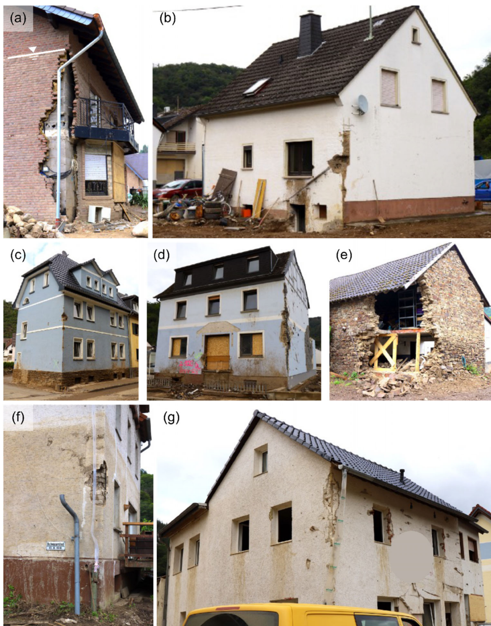
FIGURE 14 Damage and partial failures caused by the impact of floating debris, below the water-mark. (a) Dernau; (b) Altenahr; (c, d) Kreuzberg; (e) Schuld; (f) Brück; (g) Kreuzberg.
