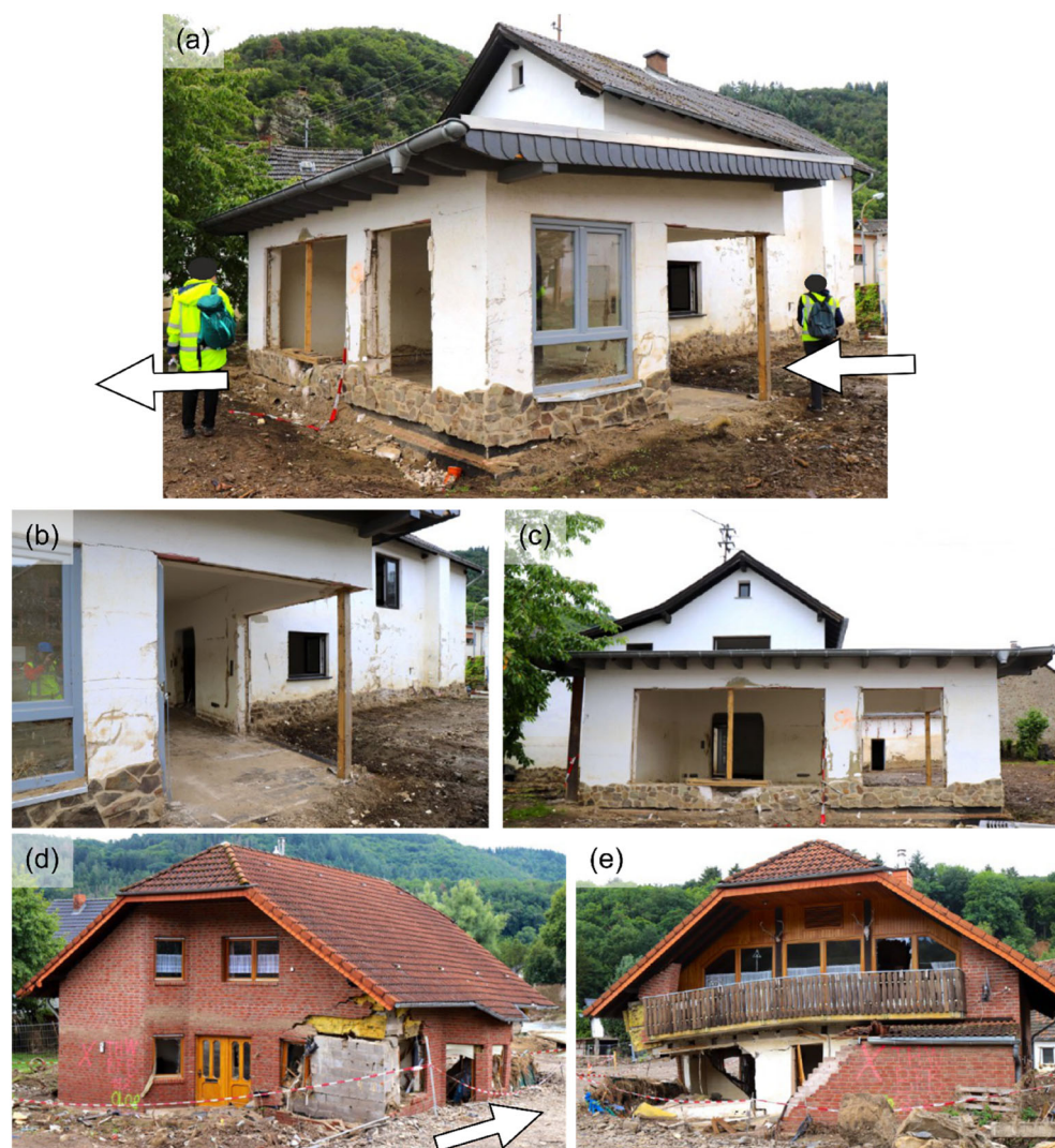
FIGURE 17 Building damage associated with the failure of single elements: (a–c) failure of a pillar in Schuld, likely associated with the debris reported inside the structure (removed, hence not visible in the picture); (d) wall tilting forward and (e) column missing at the corner in Insul. Red arrows indicate the suspected flow direction.
