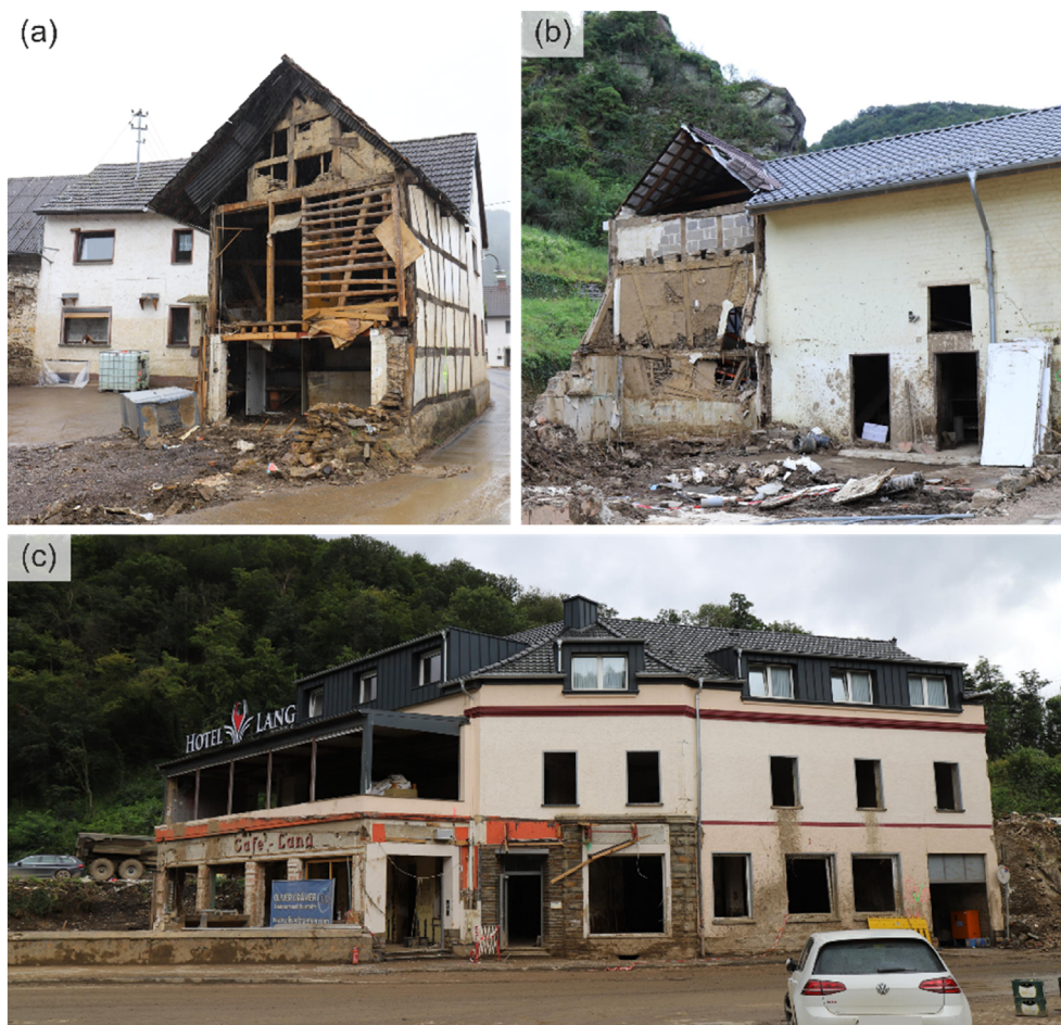
FIGURE 10 Failure of traditional half-timbered structures due to flood loading in Schuld (a) and in Kreuzberg (b) while (c) shows a modern construction in Altenahr, with a concrete structure that sustained flood loading.
