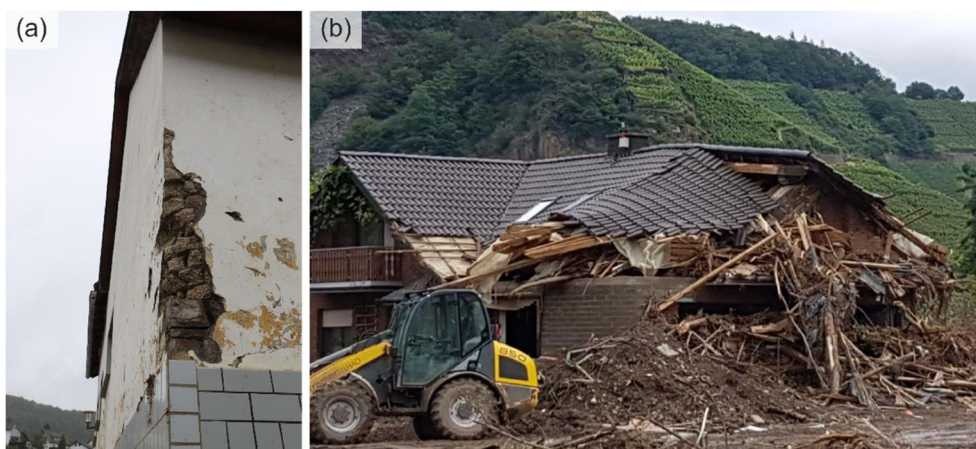
FIGURE 12 Damage associated with debris (a) marks on buildings by debris impact (Schuld); (b) debris damming around a building (Dernau).
