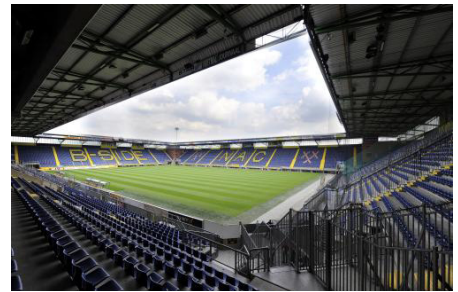
The light roof can be dismantled if desired. An engineer will have to investigate of how to put it back on its place when the extra grandstand isn't necessary anymore. This is also the case for all upcoming roofs of the stadia.
