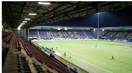
Also here a conflict can be observed between the sight lines of the extra structure and the current roof.
