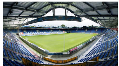
Again, also the roof must be demounted and after that if desired, put back on again.
