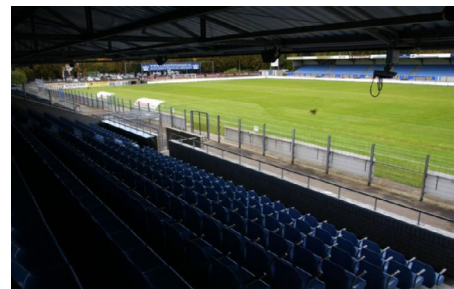
Here is also a light steel cantilevered roof structure visible.
