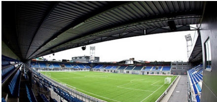
Also here, the roof is an obstruction but it seems that is can easily be dismantled.
