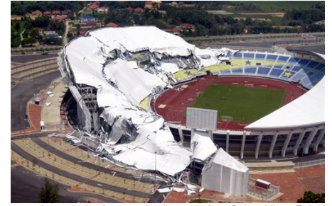
An analysis after a roof collapsed of the Sultan Mizan Zainal Abidin Stadium in Malaysia concluded that inappropriate materials and design were two factors why the accident happened. The wind took care of the fatale movement in the structure.
