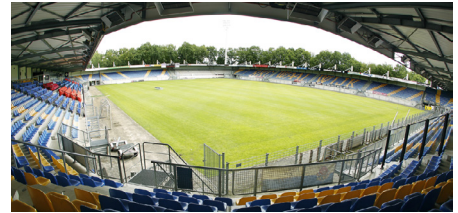
Also here, the steel roof structure must be dismantled to enable viewing lines from the extra stands.
