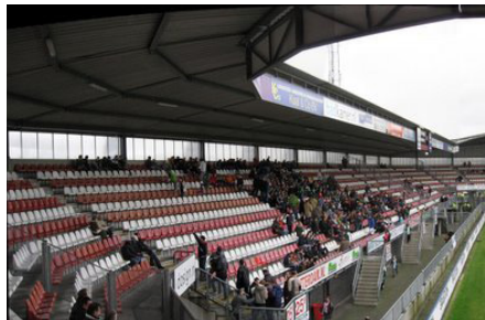
Steel cantilevers must be made into temporary ones.
