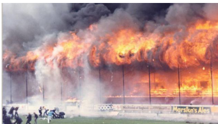
The great fire in the Bradford stadium happened after cigarette ignited a collection of trash under the stands. The disaster was live on TV, and in just a few minutes the whole grandstand was on fire. 56 people died, and over 200 got injured.
