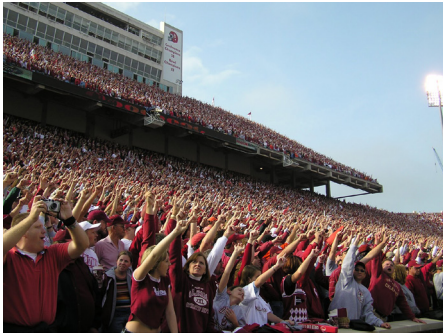
Forces not only have to be carried in vertical direction. Movements of the crowds will also cause in horizontal forces. That is why grandstand structures should be braced properly.
