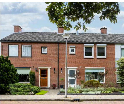
Figure 3.1: Example of CC1 building (Waard, 2023)
