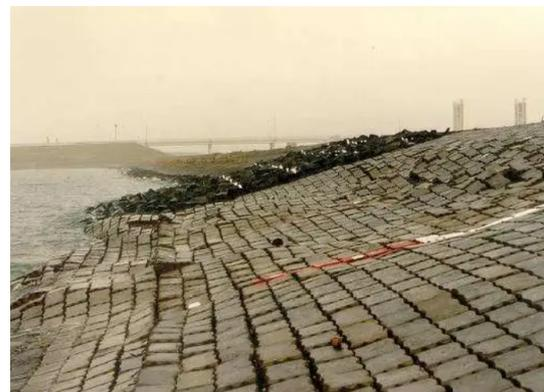
Figure 2.12: Failure of concrete mattress (Pilarczyk & Klein Breteler, n.d.)
