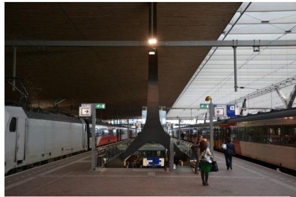
Fig 3. Roof above platform 3 and 4
