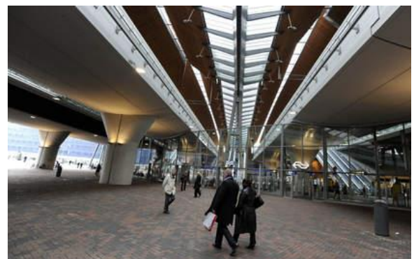
Fig 38. Glass façade that marks the station
