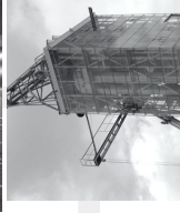
New facade elevator tower
