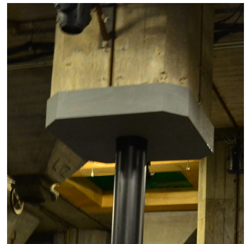
Connection covered with plywood
