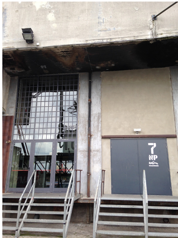
Left; New entrance - Right; closed facade with concrete plaster
