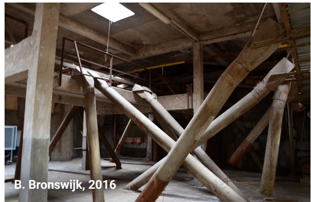
Tubes distribution system attic Stok
