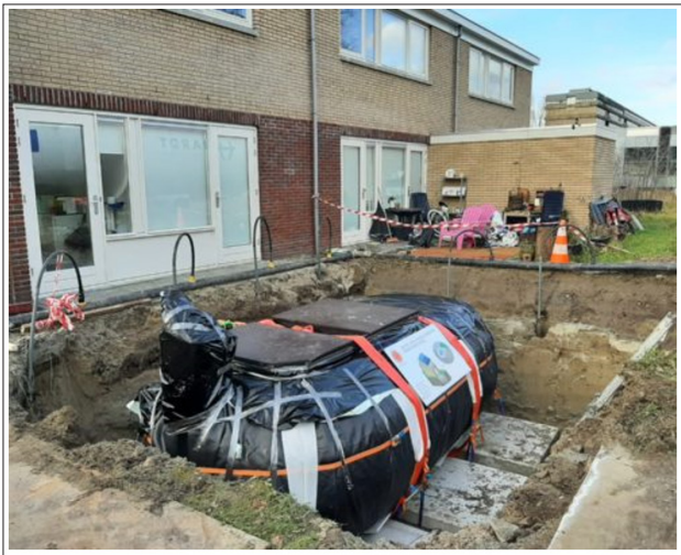
Figure 12: Image of the installation of a Borg-Buffer in a garden at the Green Village
