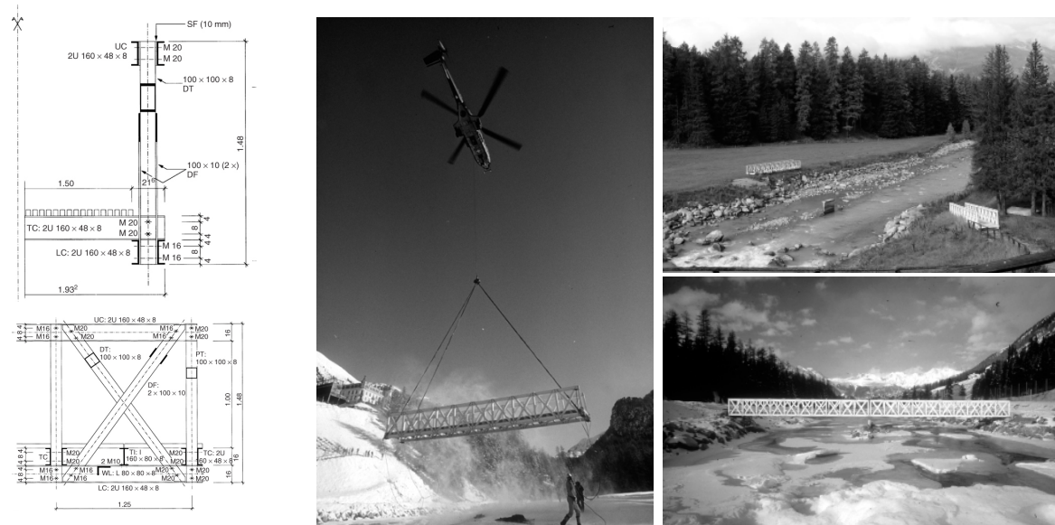
Figure 5.3: Fibre-reinforced plastic temporary footbridge
