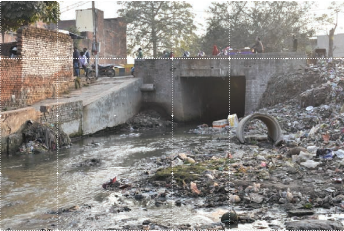
Fig 3.27: Assi nalah which originates within the city flowing as a sewage drain due to inefficient sewage, defecation, urination and solid-waste disposal Source: Columbia GSAPP,2018
