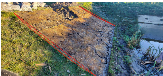
Figure 3.11: Location 2, after removal plate, red lines indicate curved shape of the subsoil
