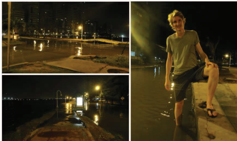
Figure 3.9 Outlets working as inlets and insufficient dike
