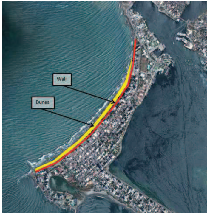
Figure 5.5 Wall with vegetated dunes
