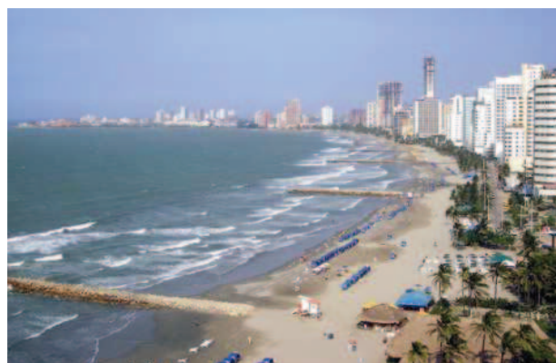
Figure 1.3 Groynes along the coast of Bocagrande
