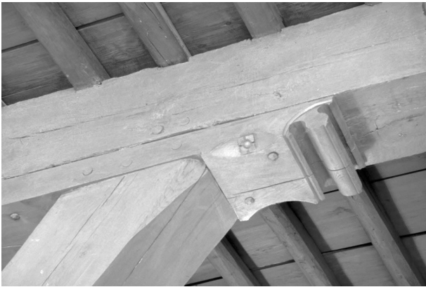
Fig. 3. Part of beam brace and decorated sole plate of Begijnhof 34 (Schoonenberg, n.d.).
