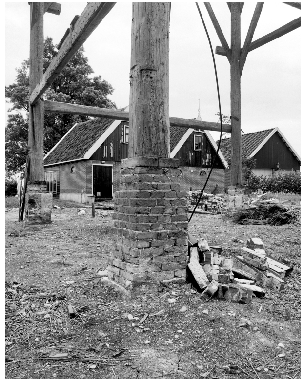
Fig. 17. Remaining central timber frame and brick footings of an unknown Stolpboerderij (Dukker, 1986).
