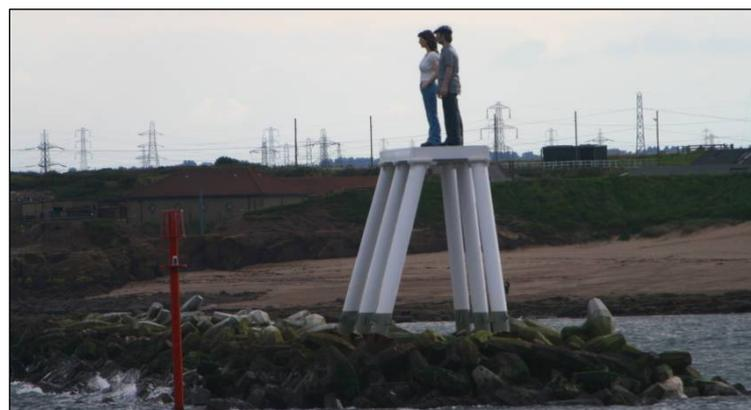
Figure 1.3 Original crest height breakwater relative to steel tube pile foundation of the monument
