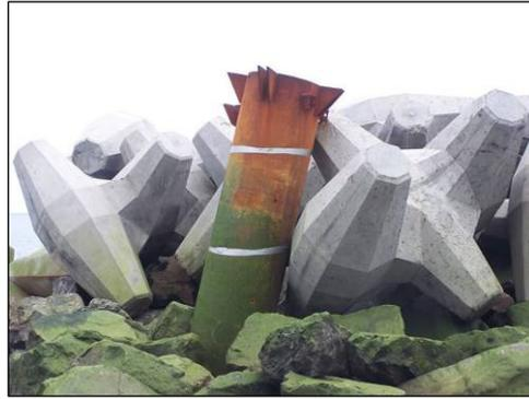
An inspection of the breakwater was carried out in June 2008 and confirmed the observed damage. Several Core-Loc units were found to have suffered damage during the structure's first winter. The number of breakages equates to approximately 1% of the total number [WAREING A.W. *et al.* 2009].
