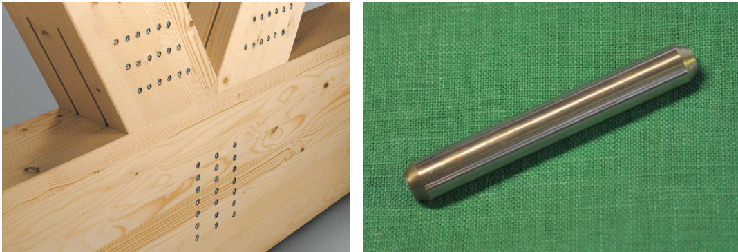
Figure 2.7: Joint with steel plates and dowels [4, 39]
