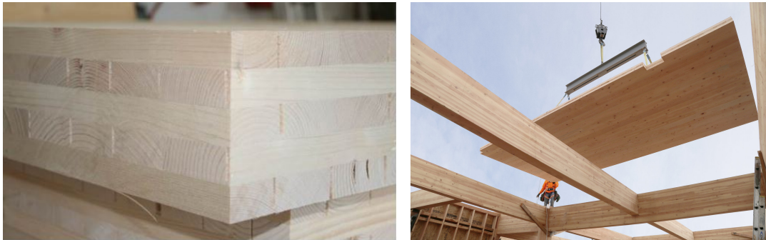
Figure 2.3: Cross-laminated timber [4, 37]
